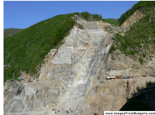
Vacha Cascade – Tzankov Kamak Hydropower Funded by EU and Austria
